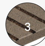
GROOVE WITH EPOXY FILLING
